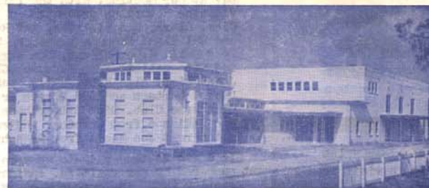
TEEN AGE CENTER BLDG., GARDENA
